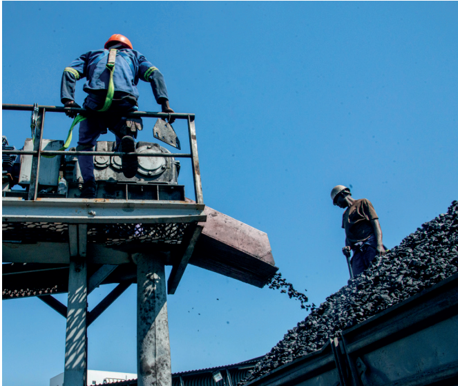
Truck loading at CHPP
