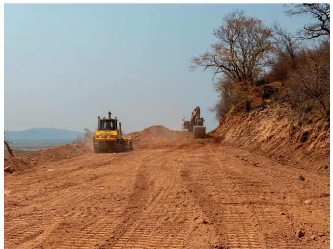
Road expansion works at Lake Kariba Pump Station
