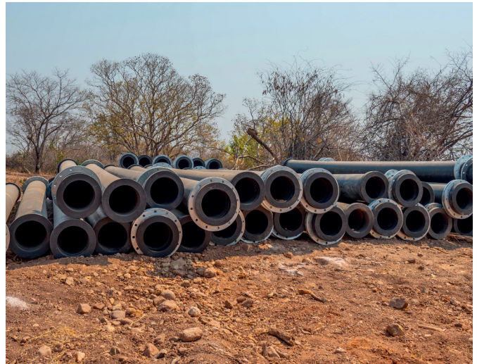
New pipes for the pipeline extension
