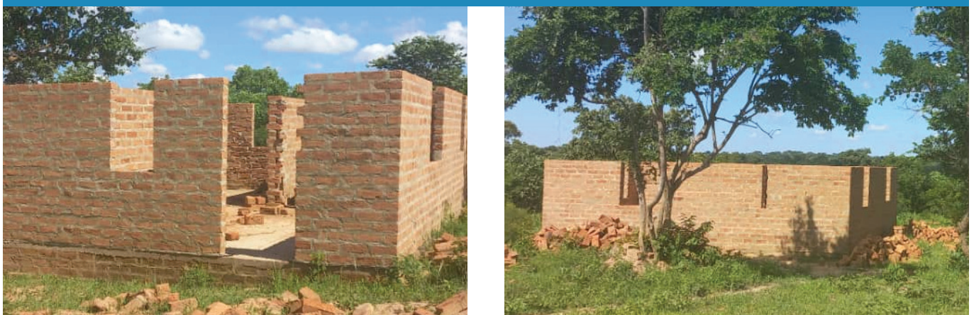
Staff Housing Unit under construction along Transmission Line.
