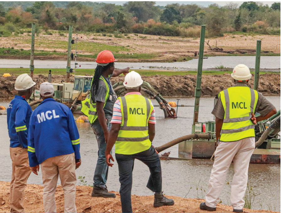
MCL team overseeing works at the dredging site at Lake Kariba
