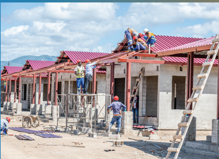
Work Continues at Phase II Construction Site
