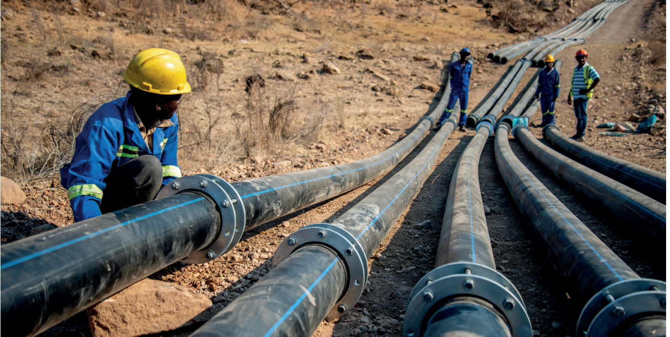
HDPE PIPES BEING LAID IN PREPARATION FOR WATERLINE EXTENSION PROJECT
