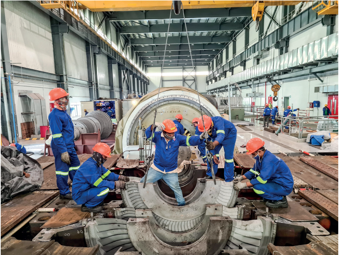
MCL ENGINEERS INSPECTING THE TURBINE
