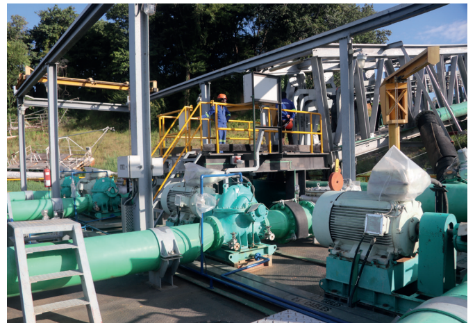
Back to Pump Station A
