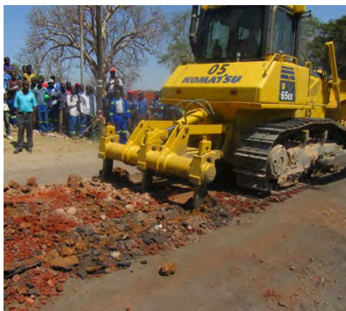
■ Dozer ripping the road to signify commencement of road works
