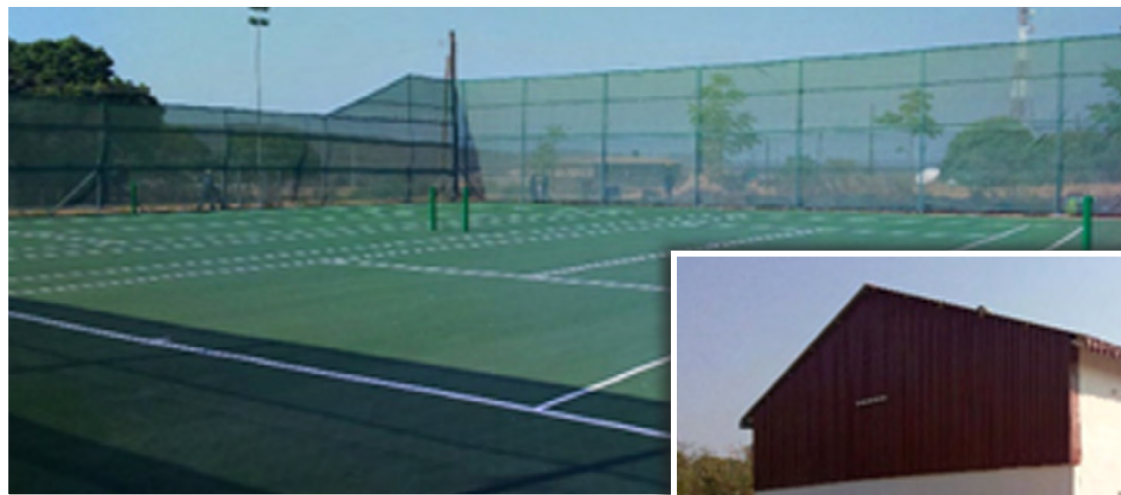
■ Newly rehabilitated Tennis Court and Gymnasium Hall
