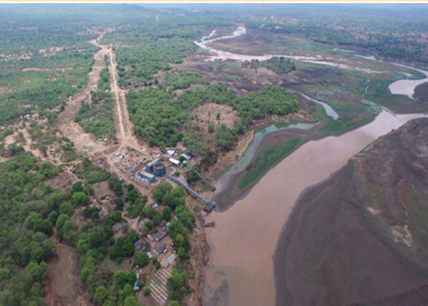
■ Aerial view of Kariba Pumping Station affected by the drought in 2015
