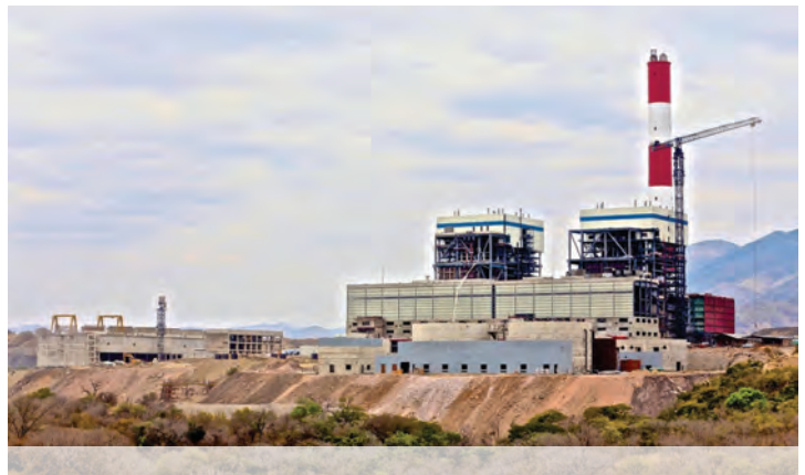
The 300MW Maamba Power Plant under Construction
