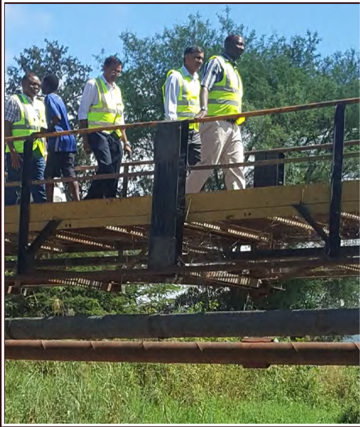
Hon. Musukwa, MP checking footbridge built by MCL to help township residents cross streams when full
