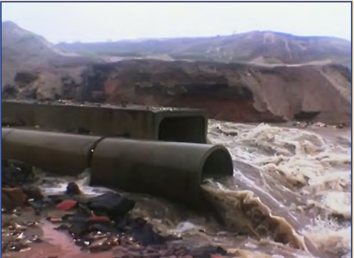
▪ Izuma B Bridge washed away due to heavy rains
