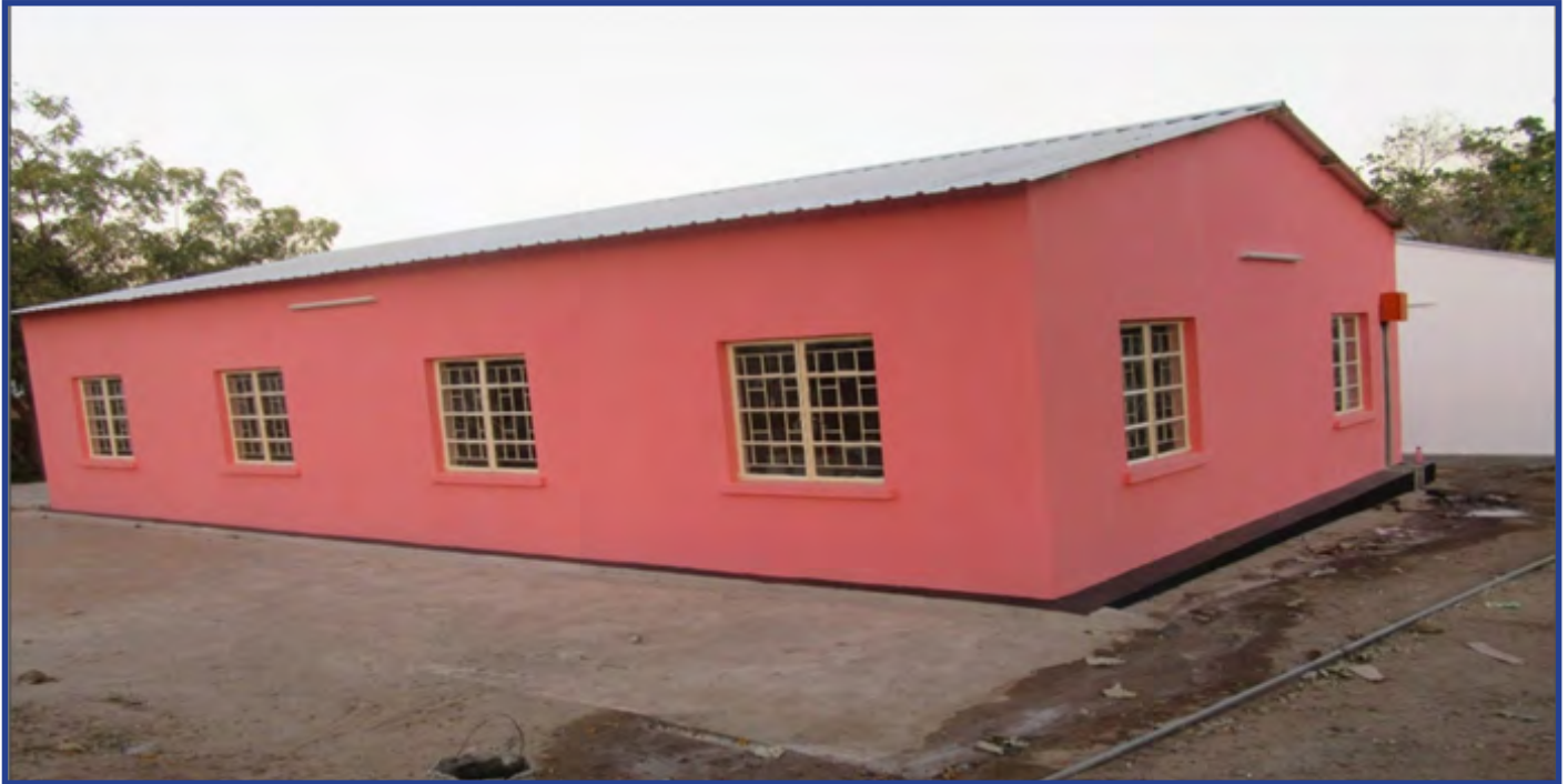
■ Rehabilitated Classroom Block at MCL's Pre-School.
