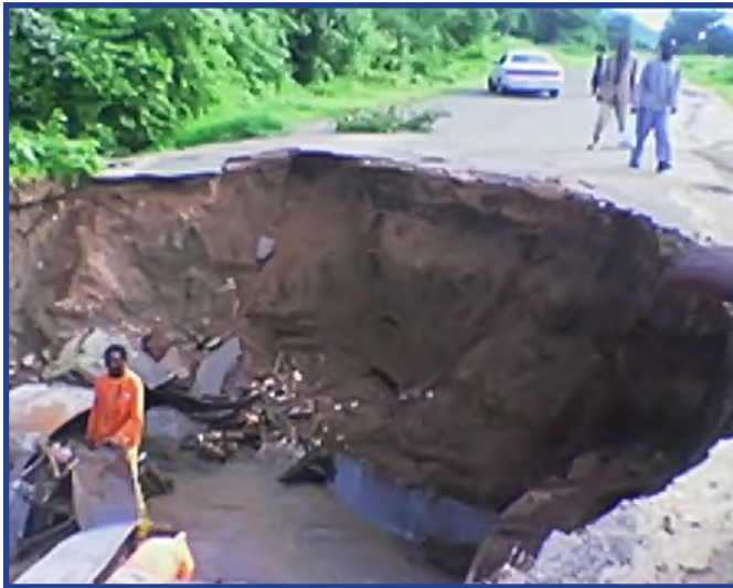
▪ Maamba – Batoka Road at Mweezya (left) and Sinazeze (left) washed away due to heavy rains
