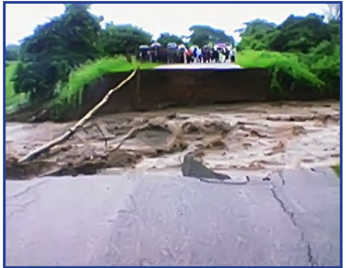
▪ Maamba – Batoka Road at Mweezya (left) and Sinazeze (left) washed away due to heavy rains
