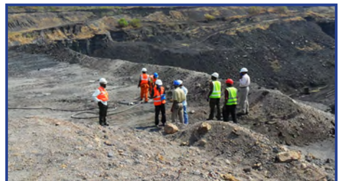
▪ Preparations for the first blast after privatization at Izuma B
