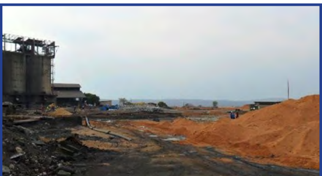
▪ Site Preparations for the new Coal Handling and Processing Plant
