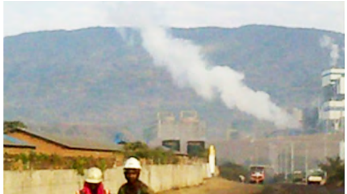
■ Steam blowing of Unit #1 piping
