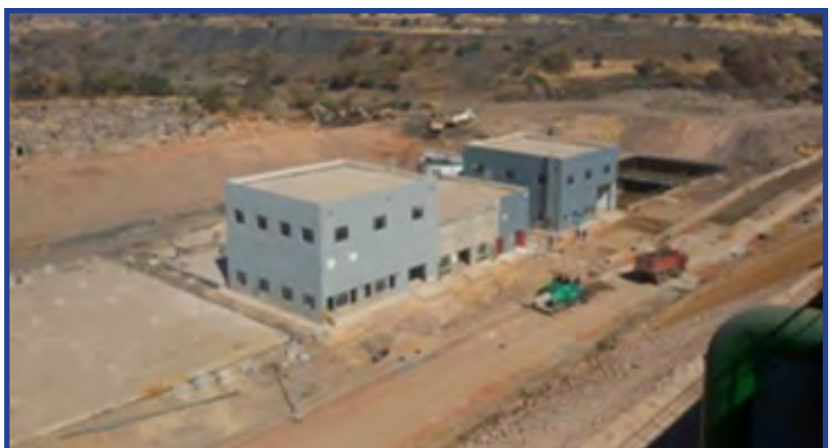
■ Industrial Waste Water Treatment Plant
