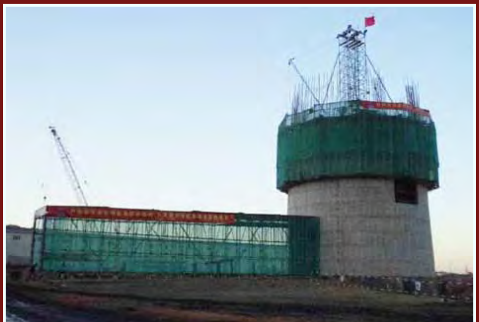
The Chimney for the Thermal Plant currently under construction in Maamba
