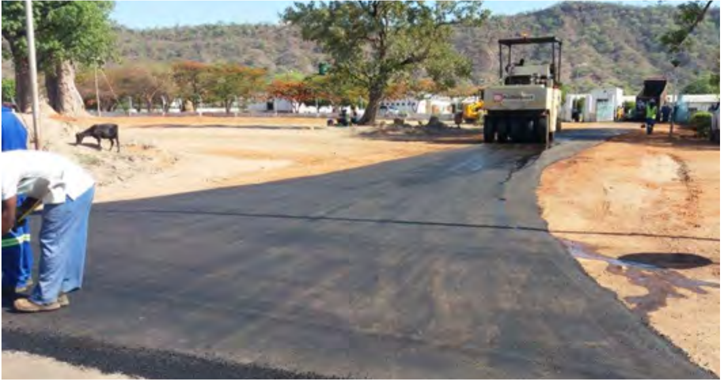
Bitumen surfacing of the road near Hospital
