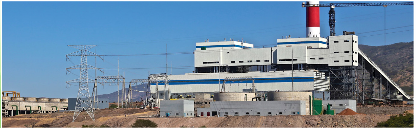
■ Maamba Thermal Power Plant
