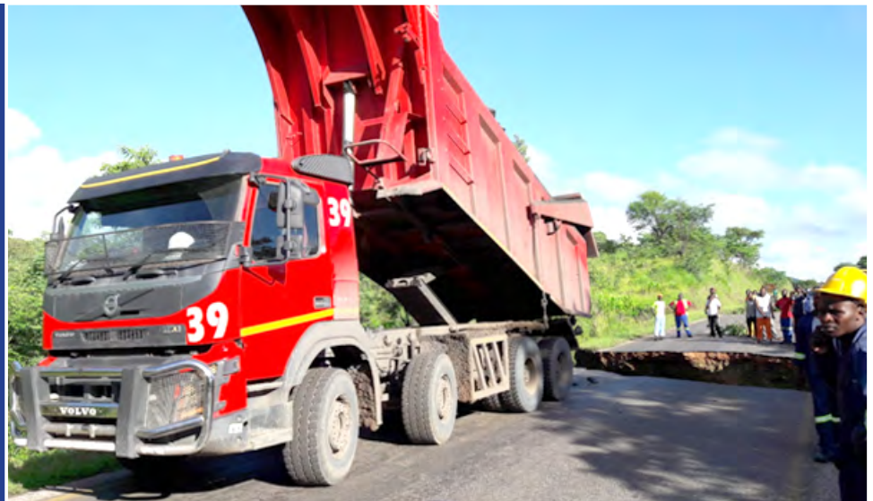
■ MCL repairing a cut away Maamba – Batoka Road on 8th February, 2017
