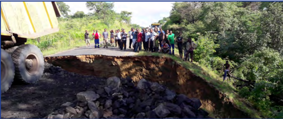
■ Back filling of the washed away Maamba – Batoka Road
