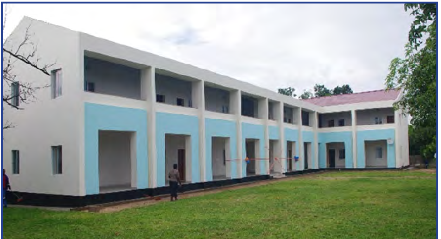
■ Newly constructed Izuma House.
