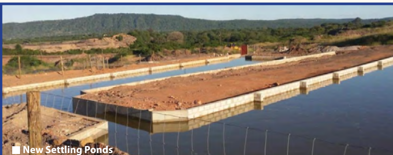
■ New Settling Ponds
