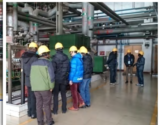
■ Site visit at Datang Shandong Electric Power Overhaul & Operation Co. Ltd
