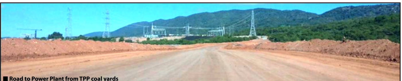
■ Road to Power Plant from TPP coal yards
