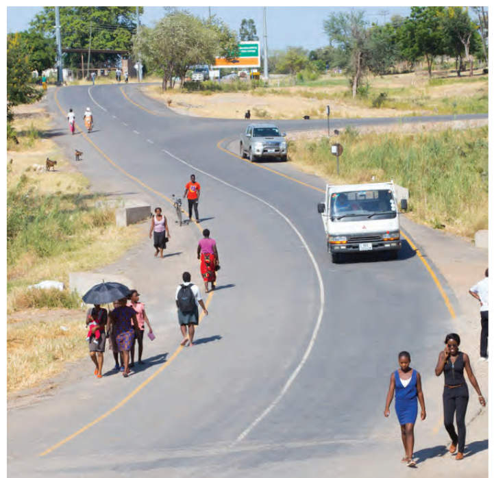
Maamba residents enjoying the safety and comfort of newly-constructed roads by MCL
