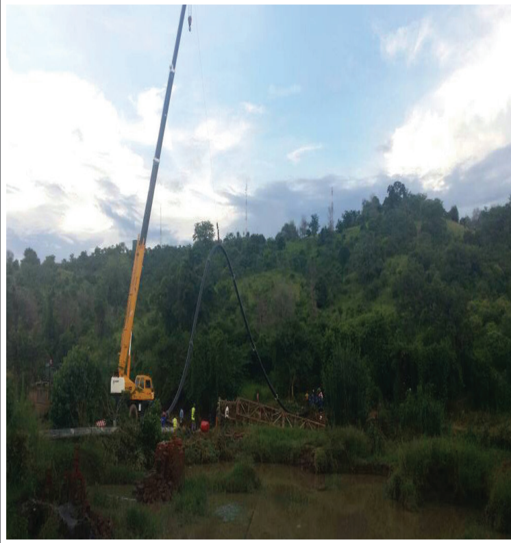
Engineers from MCL and SWASCO laying the High-Density Polyethylene pipe to restore water supply from Lake Kariba to the Water Treatment Plant in Maamba
